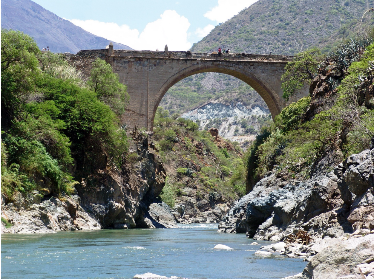
Image 1: Bridge over the River Pachachaca, outside Abancay, Peru
